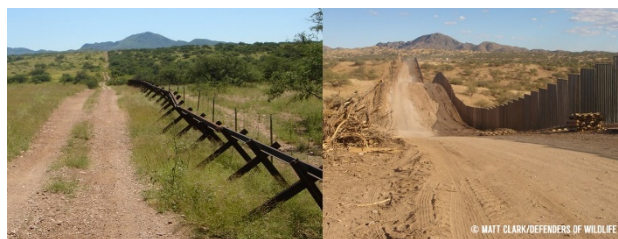
Buenos Aires National Wildlife Refuge Left: March 2007, Right: September 2007, after replacement of vehicle barrier with impenetrable barrier
